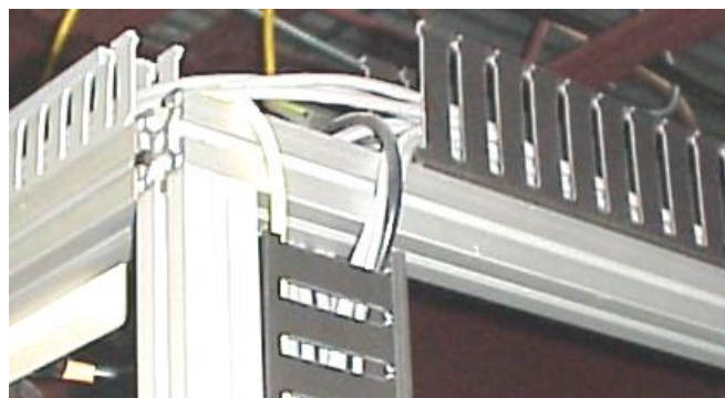
Figure 23: Wiring Channels
